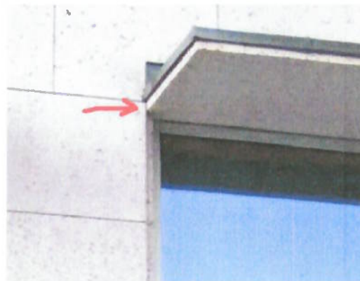
Figure 5 Stone pier to stone canopy interface. Possible contact-stress location.
